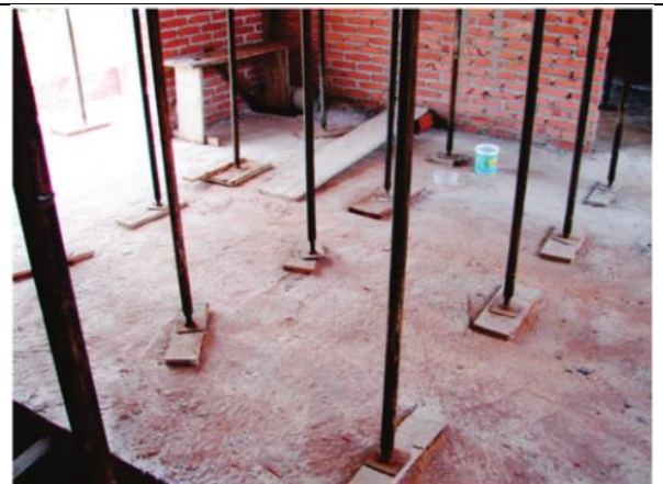
Photo 2: False work bars supported on boards
