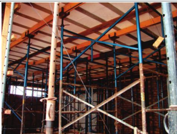
Photo 1: False work system
