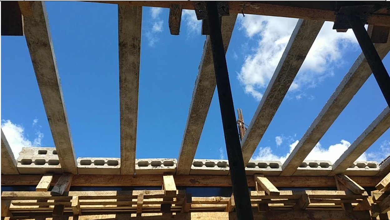
Photo 5: Lattice joists positioned ready to receive filler blocks.
