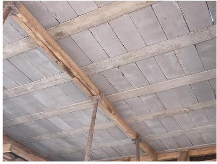
The installation of Lattice Reinforced Slab requires the use of temporary supports. In most cases, the support system will be in form of propping.
