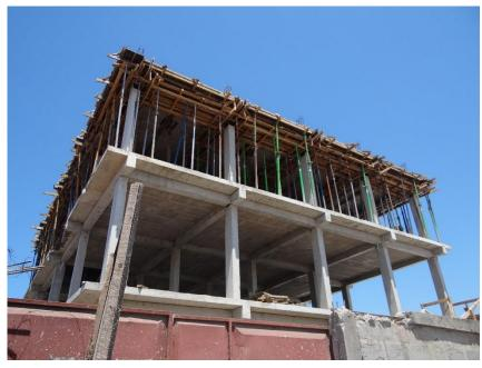
Lattice reinforced slab - system can be applied for decking both residential and multi-storeys' (floor or roof slabs).
